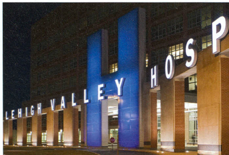
Lehigh Valley Hospital—Muhlenberg Route 22 and Schoenersville Road, Bethlehem
