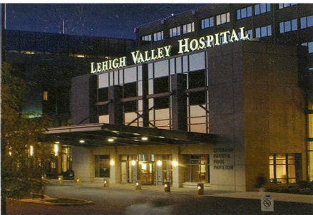
Lehigh Valley Hospital—Cedar Crest Cedar Crest and I-78, Allentown
