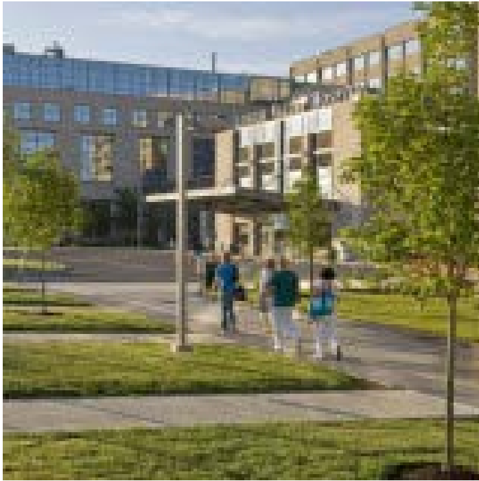
Jaindl Pavilion HVAC
