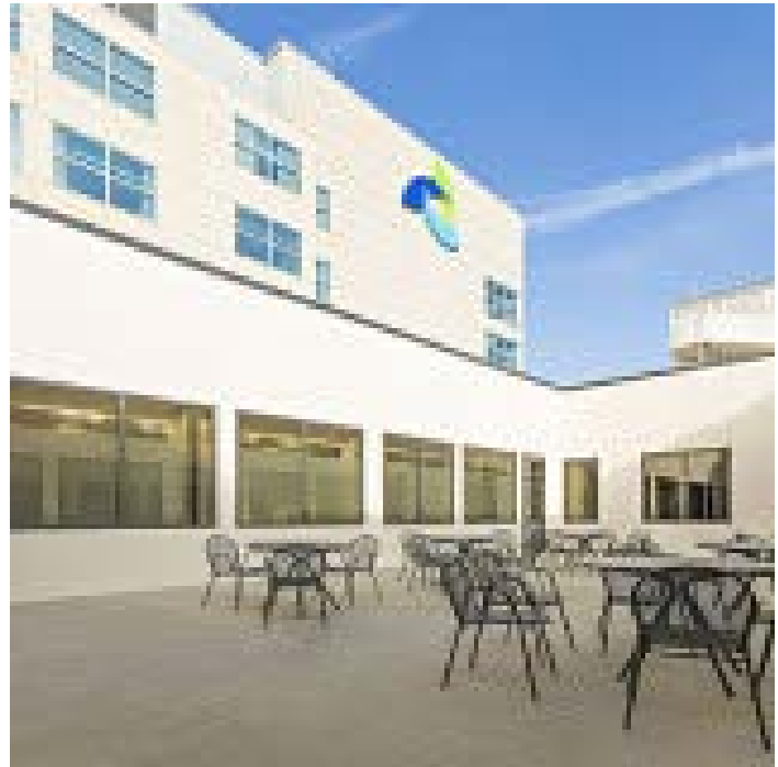
Introducing the New and Improved Anderson Courtyard
