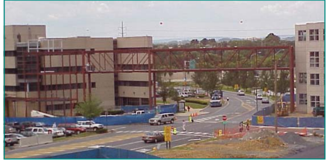
Steel trussing has been installed between the Center for Advanced Health Care with the John and Dorothy Morgan Cancer Center to support a pedestrian walkway.
