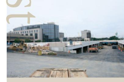
**Deck Data**—More than 280 concrete panels, weighing 5,761 tons, were delivered and pieced together to create the first of two new parking decks in front of LVH—Cedar Crest.
