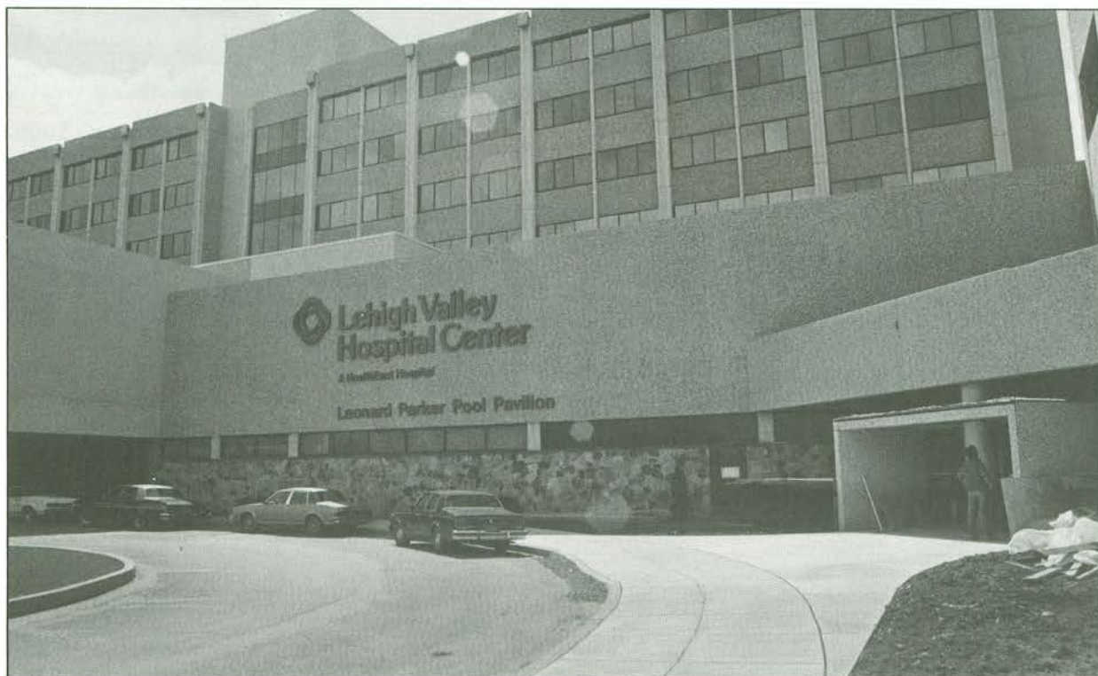
The new entrance to the right will provide easy access to the new auditorium and classrooms in the West Wing.
