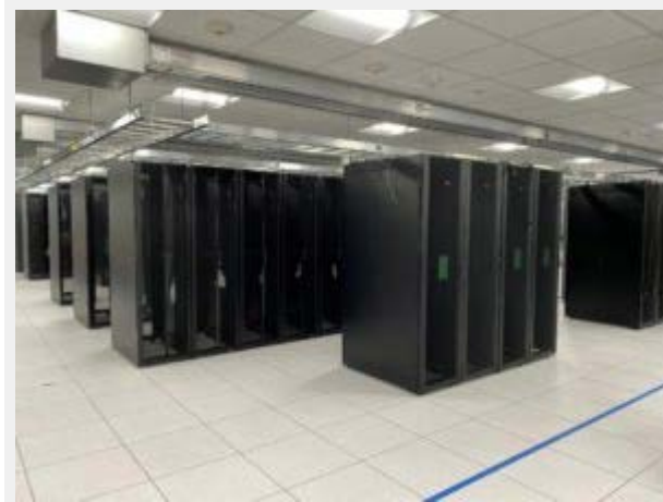
Inside one of the data centers, still under construction
